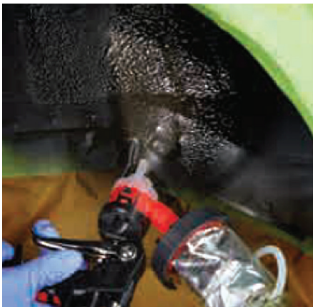
Restoring Wheel Housing Undercoating
